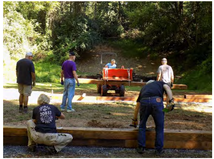
Pistol Range Repair and Maintenance
