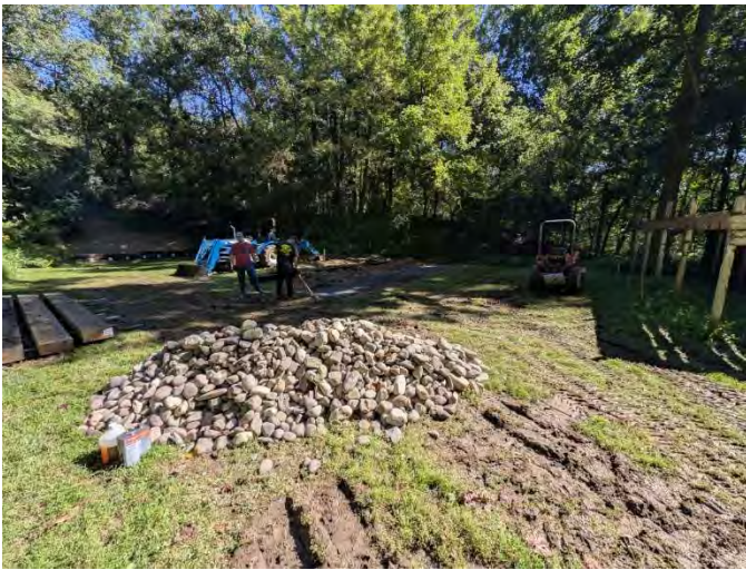
Pistol Range Repair and Maintenance
