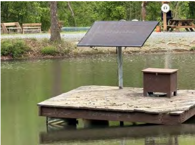
Out with the Old Lake Aerator Platform
